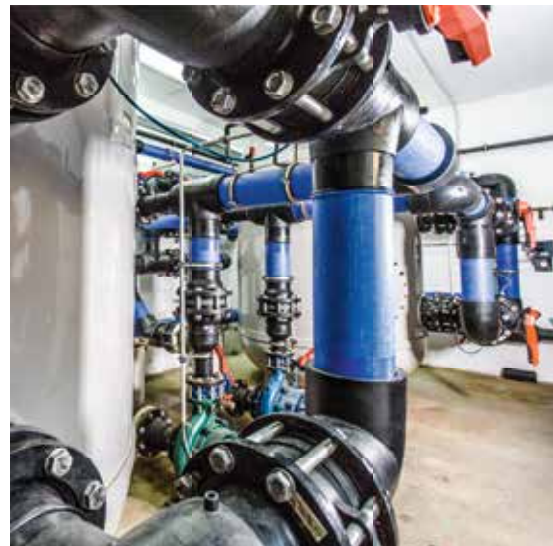
Gas installation for the fire effects of the Wodan roller coaster and water treatment system with filter station for the Atlantica SuperSplash roller coaster.
